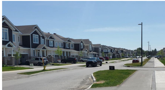
Derreen Avenue (Constructed 2023)
