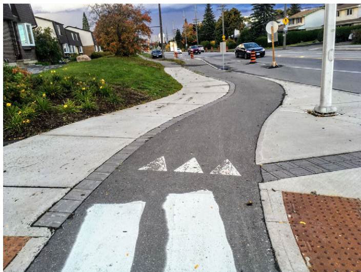
Image 5.8. Example of cycle track taper at Fisher Avenue and Dynes Road
