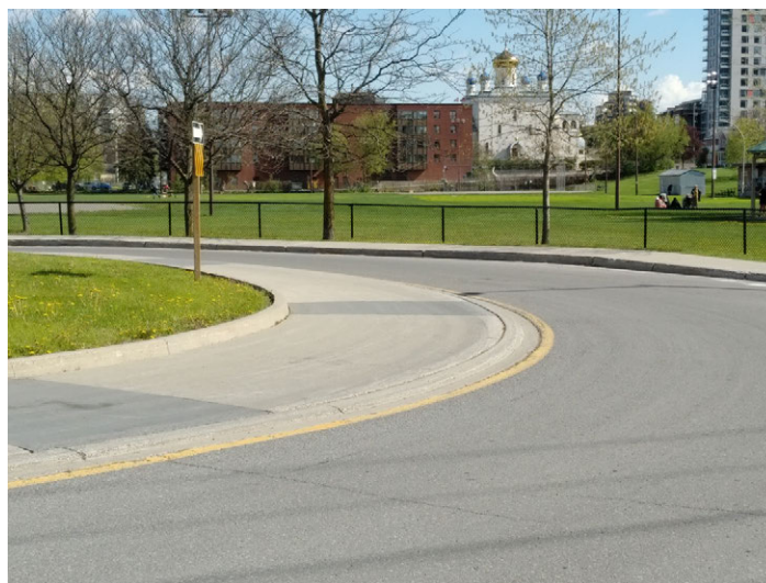
Image 6.11. Raised apron at roundabout at Bayview Station Road and Slidell Street
